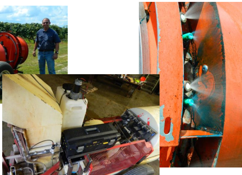
Far Right: Closeup of System 2 parallel manifolds installed in Rears sprayer
